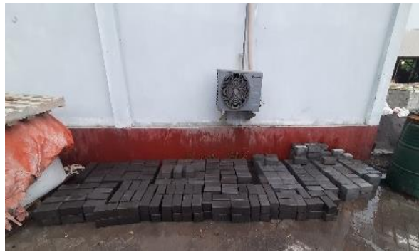
Gambar 3.17 Proses Curing Paving Block
