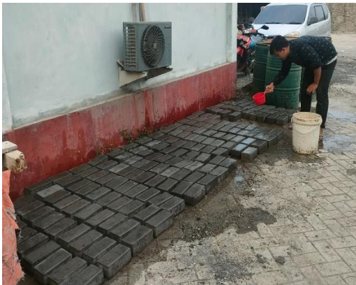
Gambar 20. Proses Curing Paving Block
