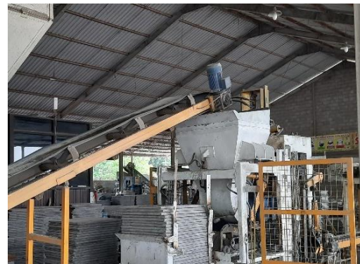
Gambar 15. Pemindahan Campuran Material kedalam Block Making Machine
