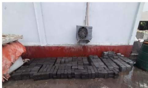
Gambar 3.17 Proses Curing Paving Block
