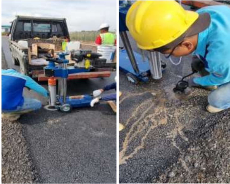
Gambar 5.3 Proses Core Drill
