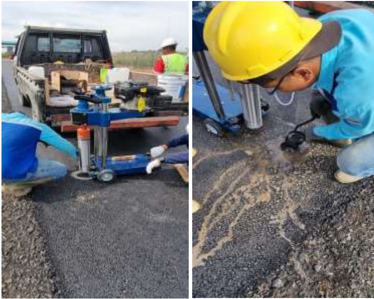
Gambar 5.3 Proses Core Drill
