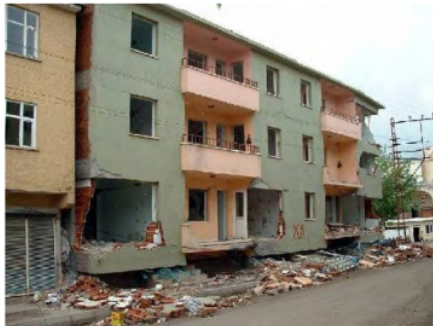
Gambar 2. Soft-storey - Gempa Bingol, Turki 2003
