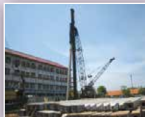
Piles Foundation for Building
