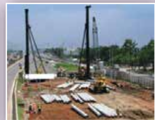
Piles Foundation for Bridges
